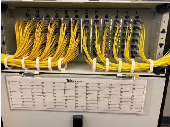
Fig. 2: Cable Termination Example Left side – 144 LCU terms demo 288 density Right side – 72 LCU terms, demo 144 density (front view)
