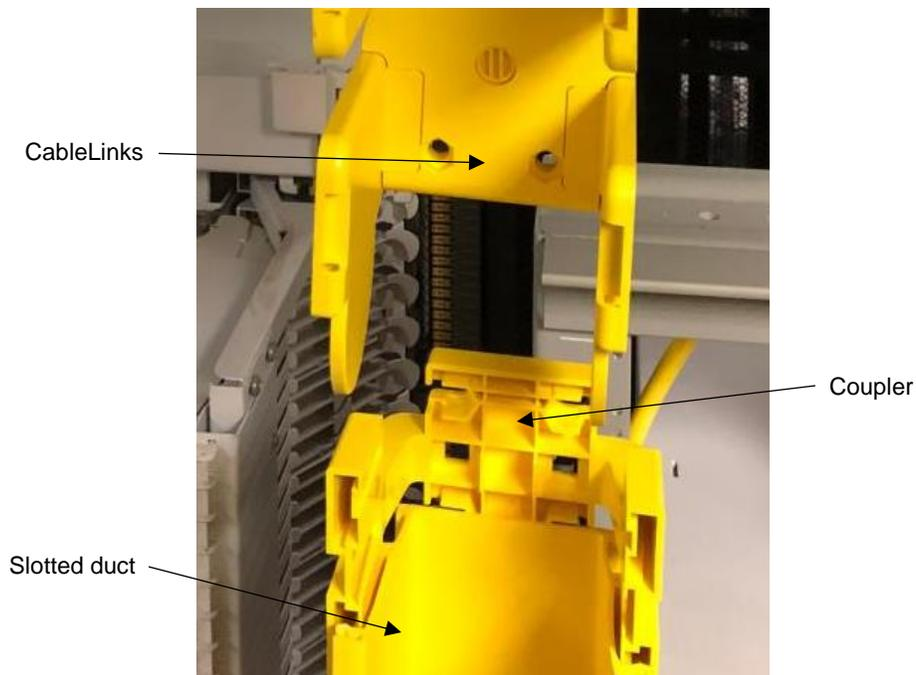
Fig. 4-61: Removing the top piece of the coupler
