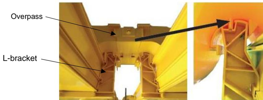
Fig. 3-127: Securing the Express Overpass to the Express L bracket
