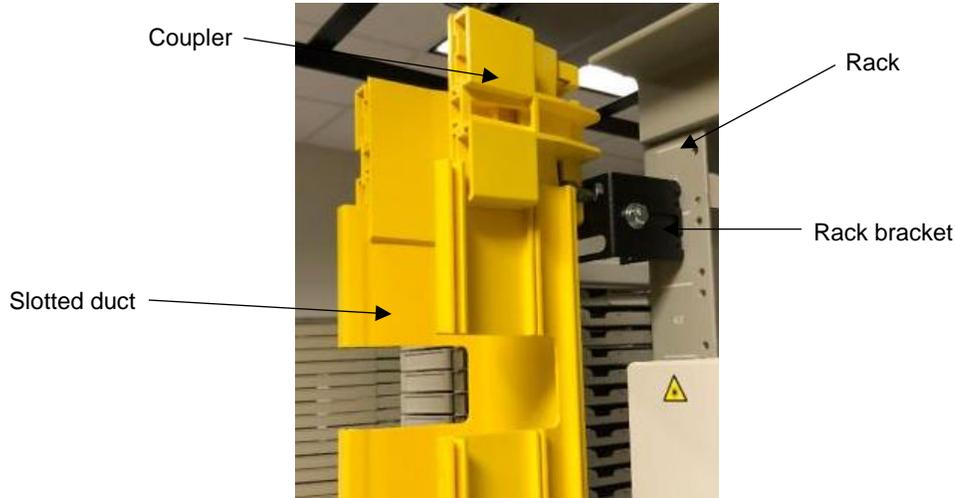
Fig. 4-58: Locking slotted duct to rack bracket with a coupler
