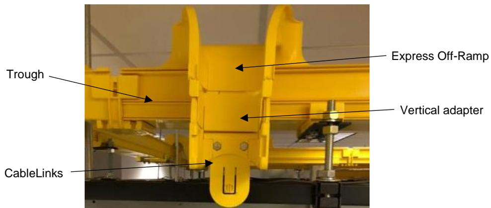
Fig. 4-59: Attaching a CableLinks module to the vertical adapter
