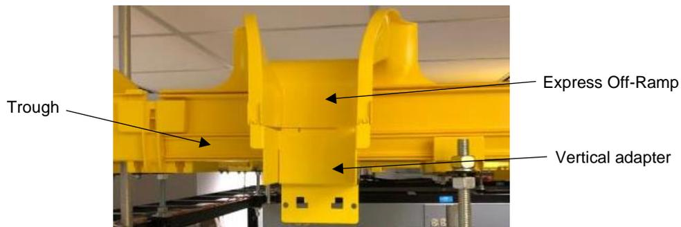
Fig. 4-52: Attaching vertical adapter to the vertical component
