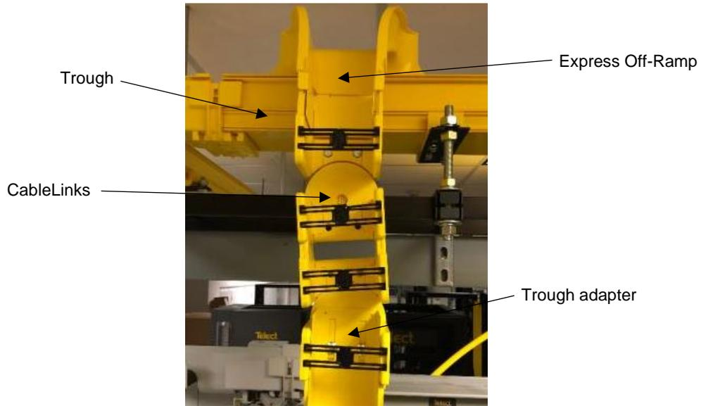
Fig. 4-64: Installing the H-shaped gates to the CableLinks modules
