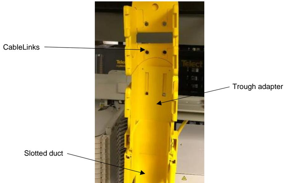
Fig. 4-62: Locking the trough adapter to the slotted duct with a coupler
