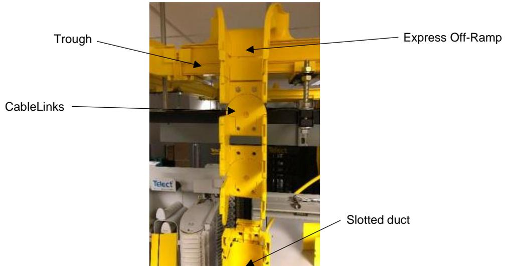
Fig. 4-60: Adding CableLinks modules
