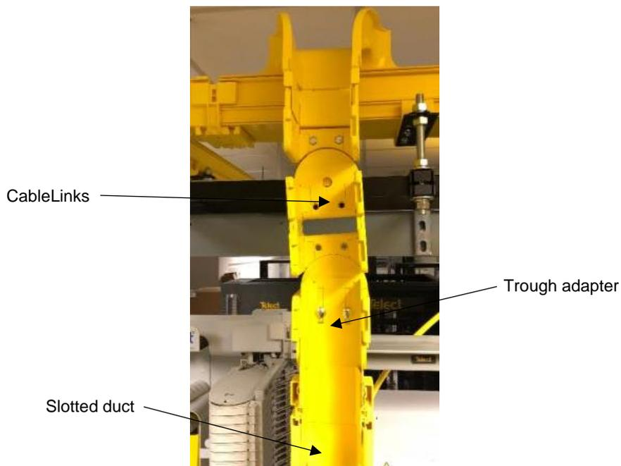
Fig. 4-63: Securing the trough adapter to the CableLinks module
