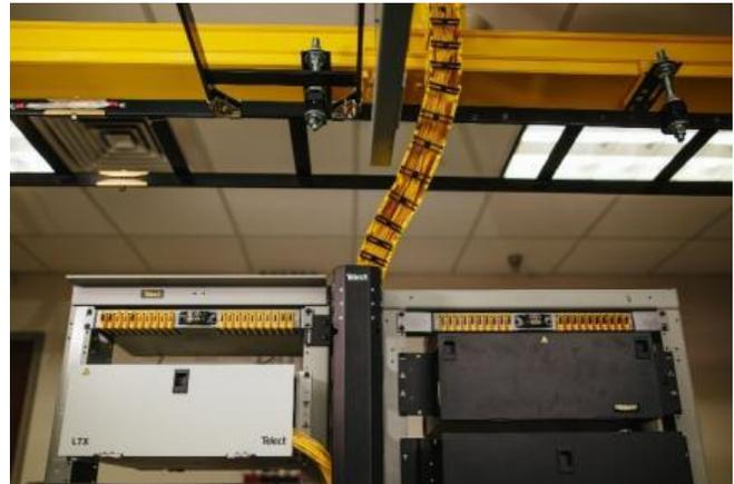
Fig. 1-19: CableLinks vertical path change
