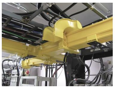
The Express series of products, particularly the Off-Ramp, feature custom-engineered support brackets that provide convenient fastening and easy re-configuration or expansion.
