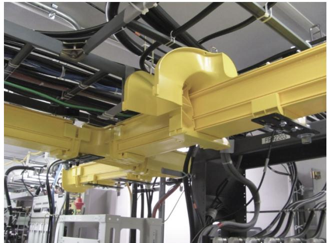
The Express series of products, particularly the Off-Ramp, feature custom-engineered support brackets that provide convenient fastening and easy re-configuration or expansion.
